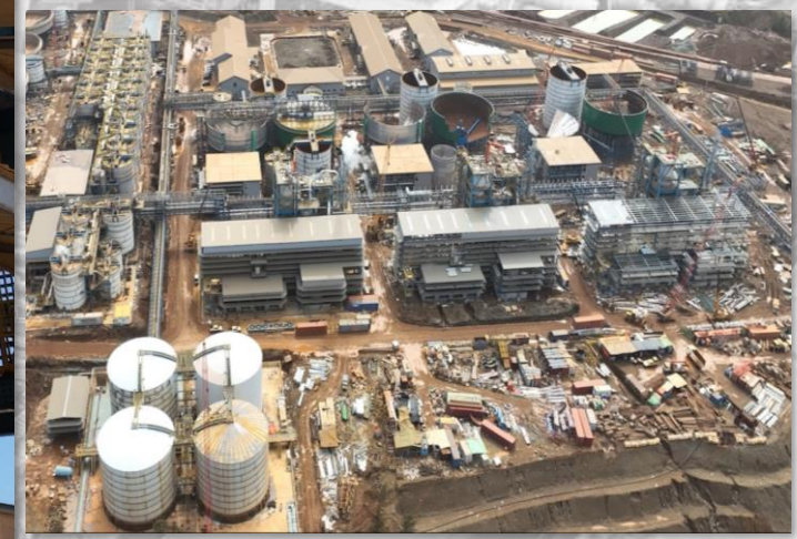
1 st 2 nd and 3 rd autoclave, 1 st 2 nd and 3 rd ore slurry storage & thickening and concentrated sulfuric acid storage tanks
